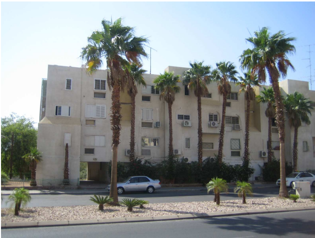
View of Apartment 1146 building on Sheshet HaYamim.
